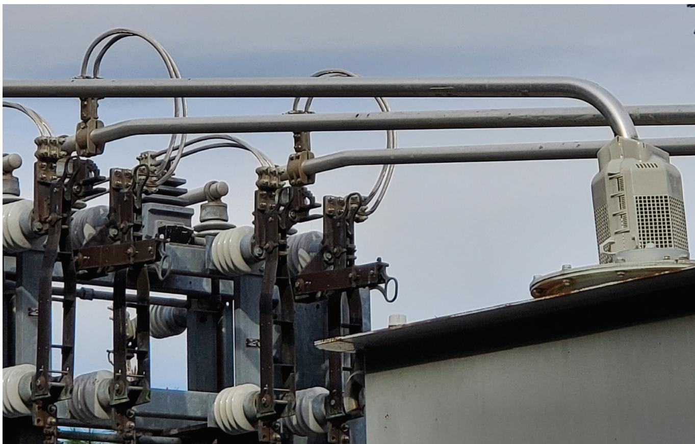
During monthly substation inspections, bullet holes were found in the overhead incoming and outgoing bus work—in a Klickitat PUD substation.
