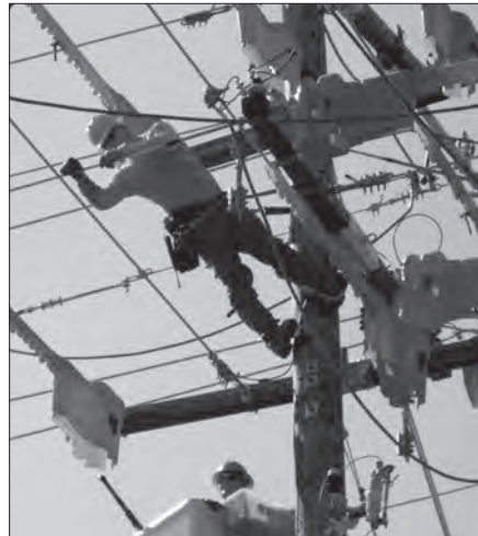
Clockwise from top, the Goldendale crew works to remove and replace broken poles on Alderdale Road during a severe windstorm. KPUD Journeyman Lineman Justen Greenwood works “out of his hooks” surrounded by cover that allows him to get close to the live power lines for a new wire installation project. TJ Lutz makes his way to an outage on Flat Top Mountain in Trout Lake via a Snow Cat.
