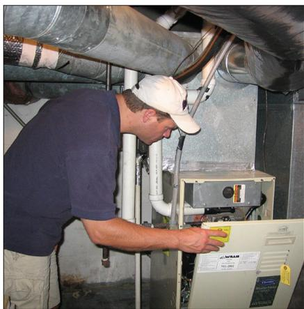
To inspect your gas furnace heating system, first turn off the electric circuit breaker, then remove the cover from the burner and control portion.
