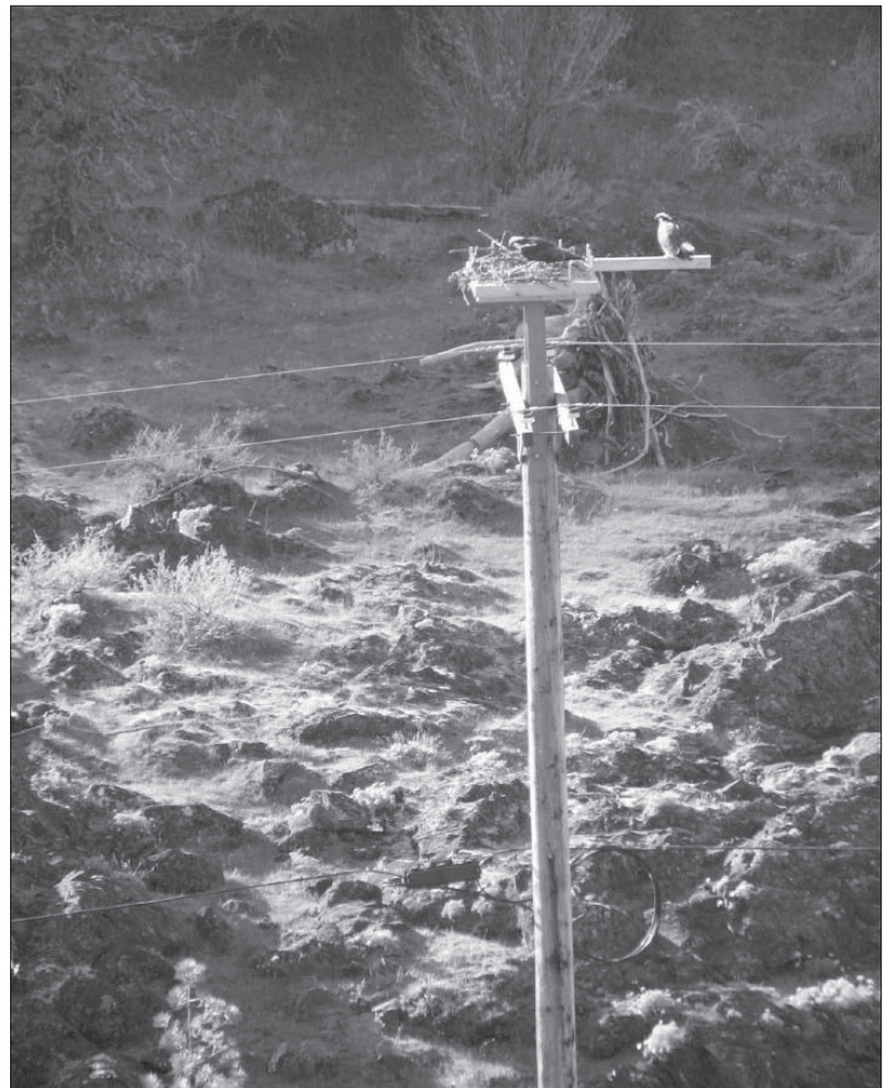
A pair of osprey occupy a nest atop a KPUD pole with a new platform along the Klickitat River.
