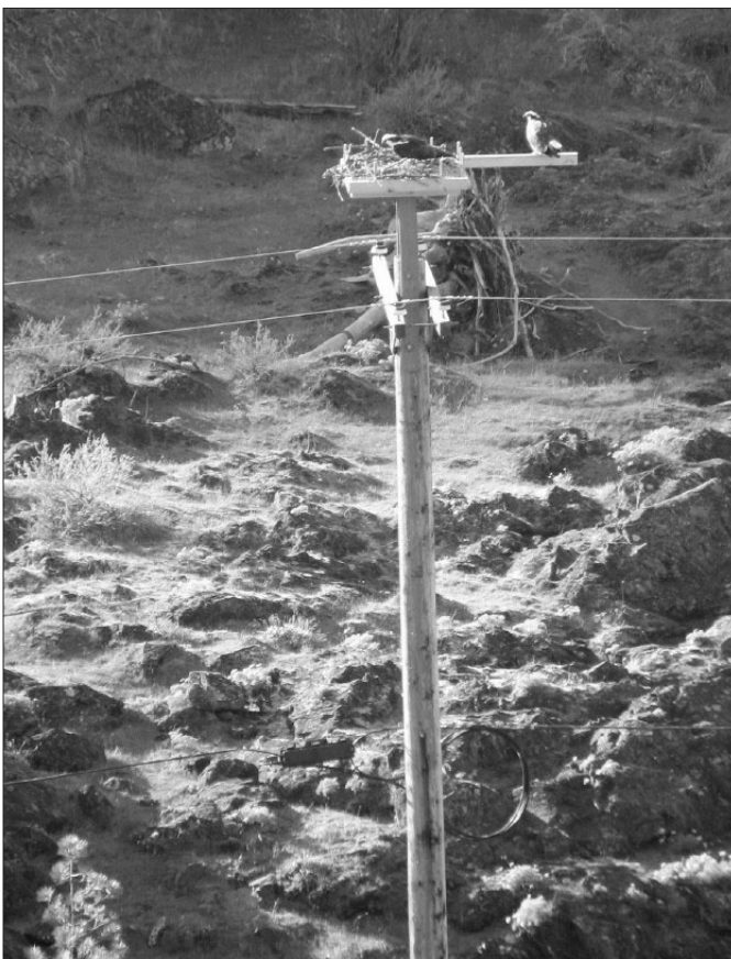
A pair of osprey make themselves at home on a nesting platform built on the top of a Klickitat PUD utility pole.
