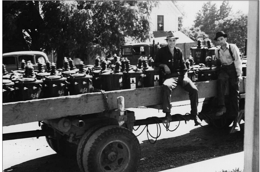
Two early Klickitat PUD employees with a load of transformers for the Trout Lake – Glenwood line.
