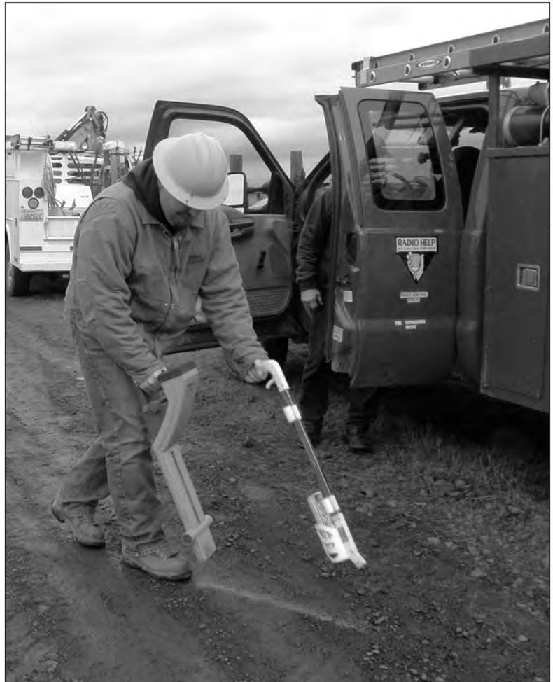
**Travis Heilman demonstrates how underground power lines are located and then marked in red paint.**
