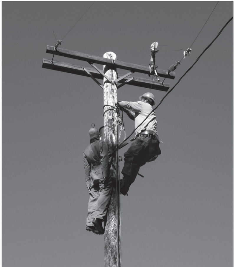
Above, KPUD Lineman Bernie Predeek ties the rescue line in position on the pole to lower Bill, the rescue dummy.
