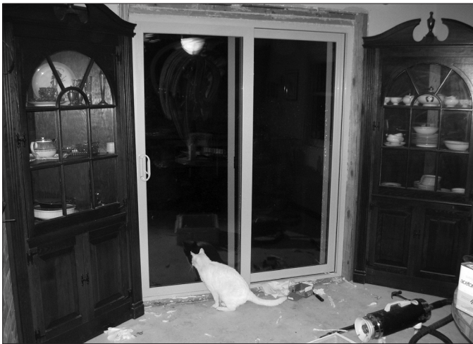
An installed sliding glass door with only interior trim still needed.
