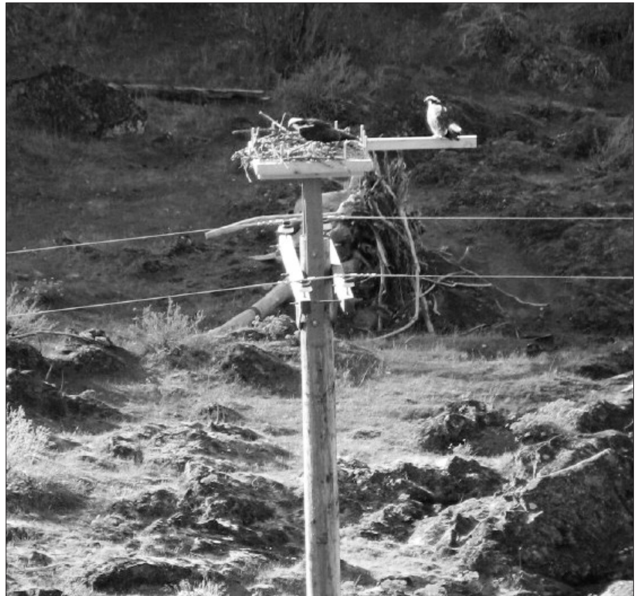
An osprey nesting platform atop a Klickitat PUD power pole has a few feet of separation from cross arms.
