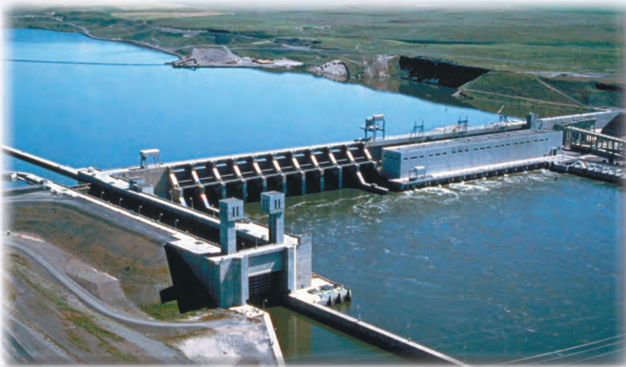
Ice Harbor Dam on the Lower Snake River.
