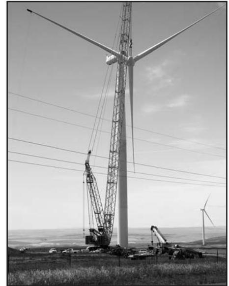
bine is complete. The nacelle, rotor and blades weigh more than 160 tons. The nacelle, alone, is about the size of a motor home—12 feet by 12 feet by 36 feet.
