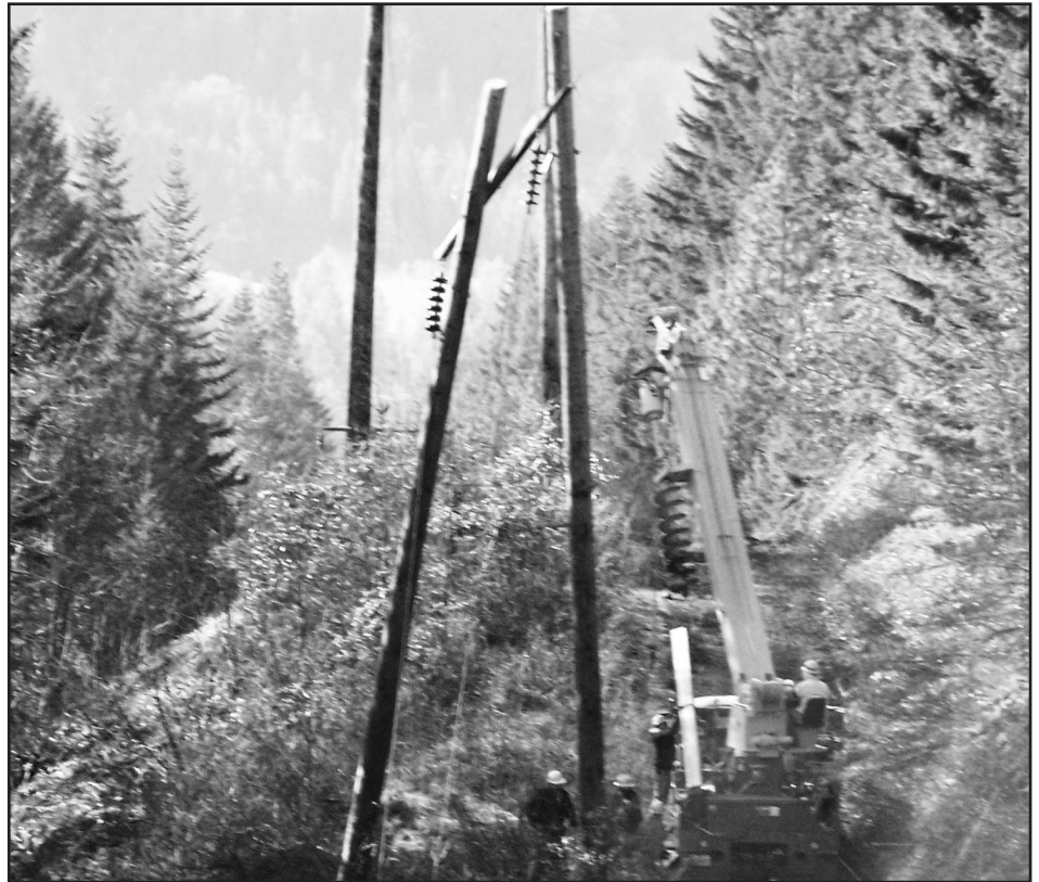
Above, KPUD crews worked day and night to rebuild damaged poles and equipment and restore power caused by the severe windstorm in December.
