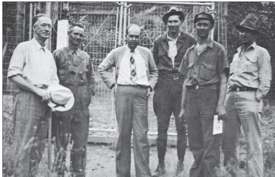
First power flowed into PUD lines in the fall of 1941, and these men were present for the occasion. Power was taken from Pacific Power & Light's substation at Condit in an exchange agreement with the Bonneville Power Administration. From left are J.S. Degman, PUD commissioner; Orville McCutchan, PUD lineman; Emmet E. Clouse, PUD manager; Jack Barbiur, Bonneville lineman; Lawrence McCuiston, PUD lineman; and Otto Reeves, Bonneville groundman.
