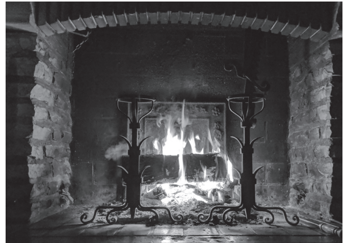
Burning wood produces radiant heat, which feels great if you're near the fire. But it can also send large amounts of room air up the chimney.
