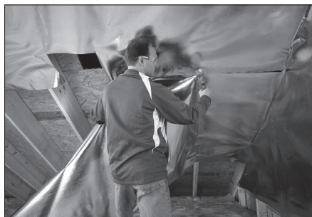
Radiant heat barriers often look like aluminum foil. It only reflects radiant heat toward an air space of at least 1 inch.
