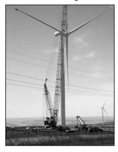
bine is complete. The nacelle, rotor and blades weigh more than 160 tons. The nacelle, alone, is about the size of a motor home—12 feet by 12 feet by 36 feet.
